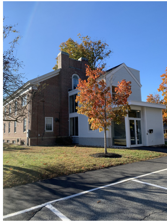
Pilgrim House (Church office, community meeting space, and Church school) Renovated in 2018 with elevator and new entry.
