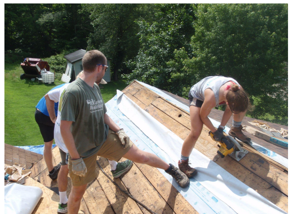
Peace Youth repairing roof. Philippi, WV
