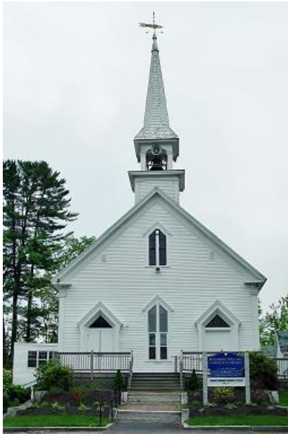
Erected in 1879, recently re-sided
